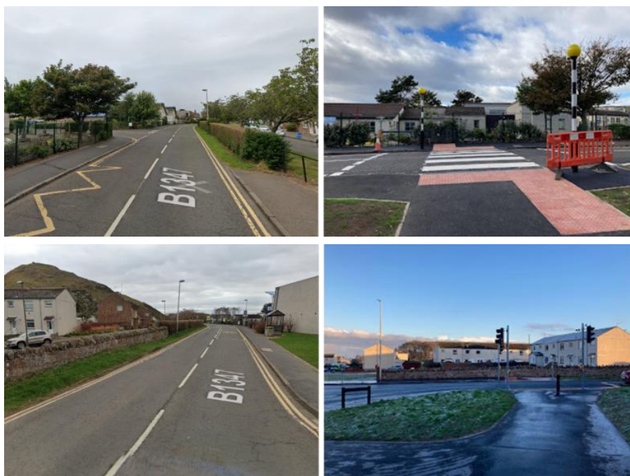
Figure 16: Before and after photos of the zebra crossing constructed near the schools
